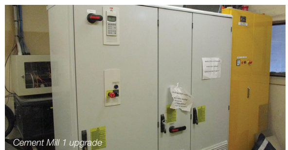
Cement Mill 1 upgrade
