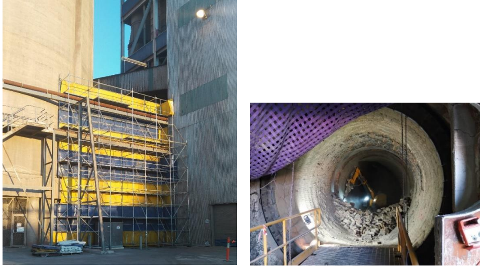
Photo of noise attenuation barrier and pneumatic breaker in the kiln
