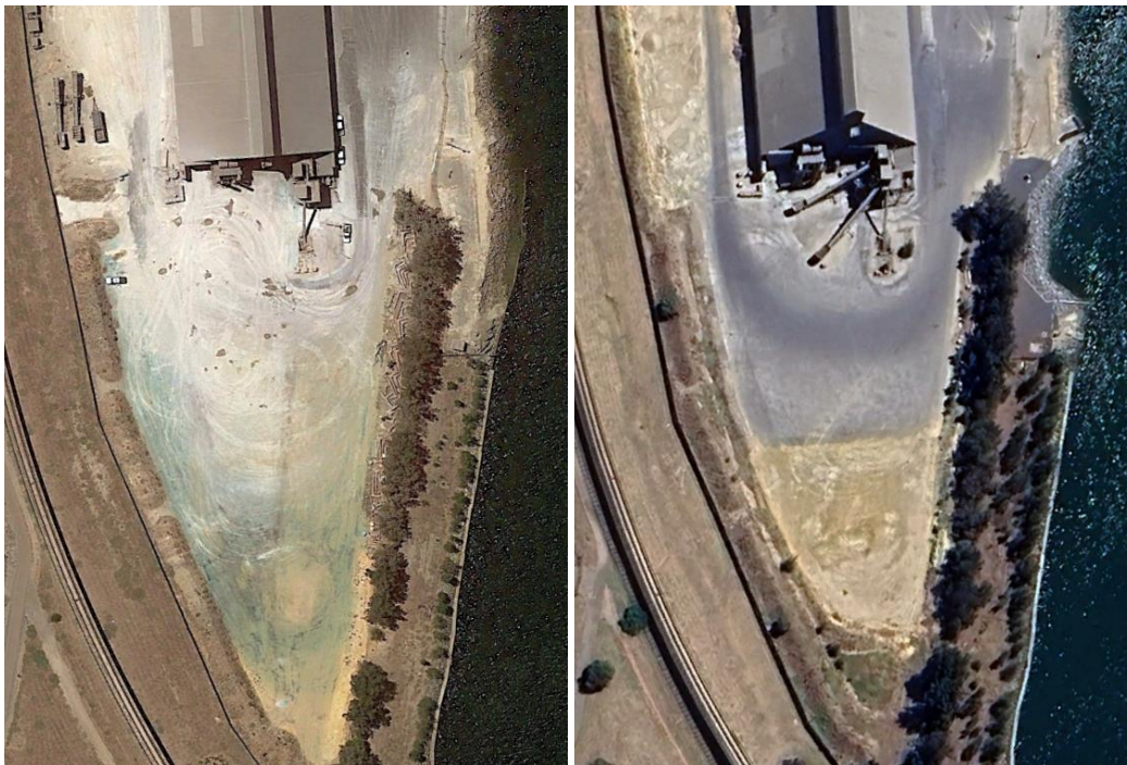
Figure 1 Area south of clinker blend building before (left) and after (right) sealing
