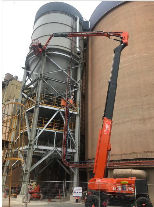
Photograph of silo nearing completion of installation
