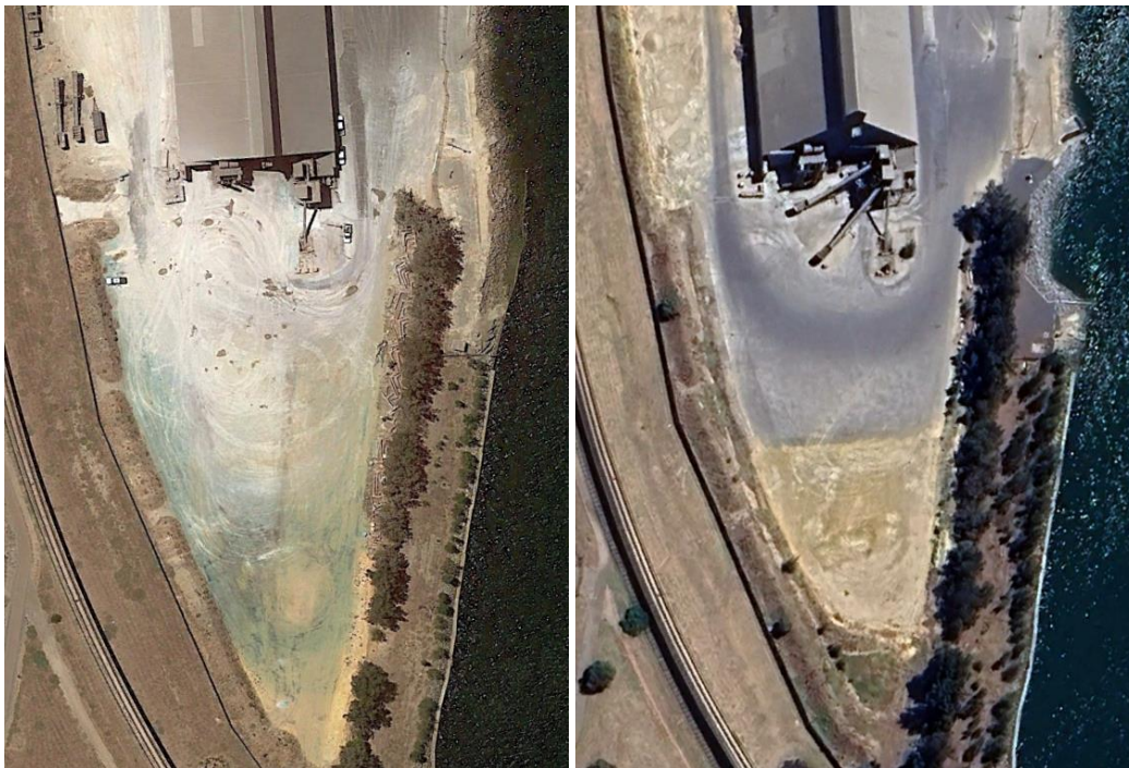
Figure 1 Area south of clinker blend building before (left) and after (right) sealing
