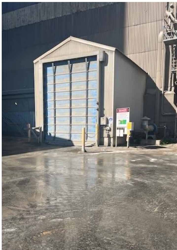
Clinker shed air knife and rapid raise door
