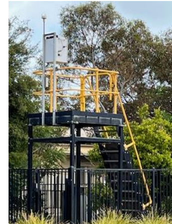
Typical air monitoring station
