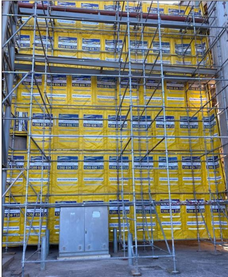
Figure 4 Temporary noise barrier installation during shut down period
