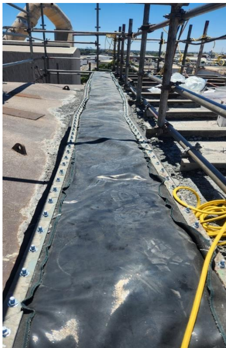
Heat exchanger inlet expansion joint replacement
